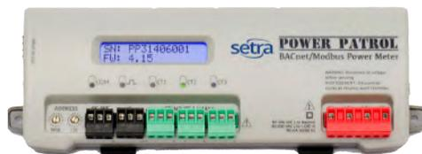
The Setra Power Patrol is every electrical contractor's dream. The Revenue Grade networked 3-phase power meter works with Rogowski Coils and has a small enough form factor to be mounted inside or outside of the panel using either mounting tabs or the DINrail clip making it the easiest installation in the industry.
