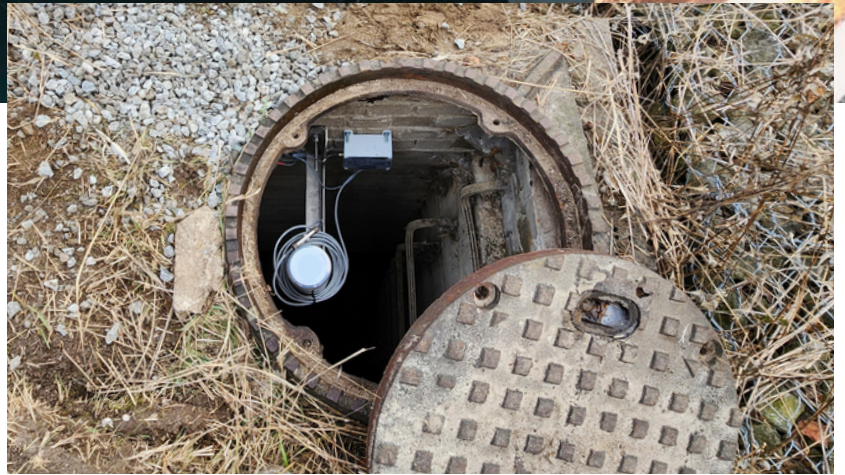
Figure 1: ABM non-contact radar level sensor and cellular gateway installed in a manhole.
